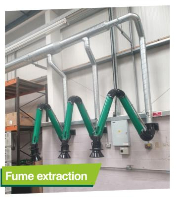
Fume extraction can range from simple welding extract arms through to highly specialised chemical-resistant containment systems.
